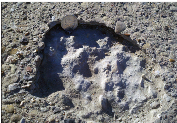
Pit in concrete
